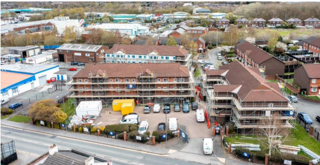
Stadium View on the Peasley Cross site undergoing refurbishment
